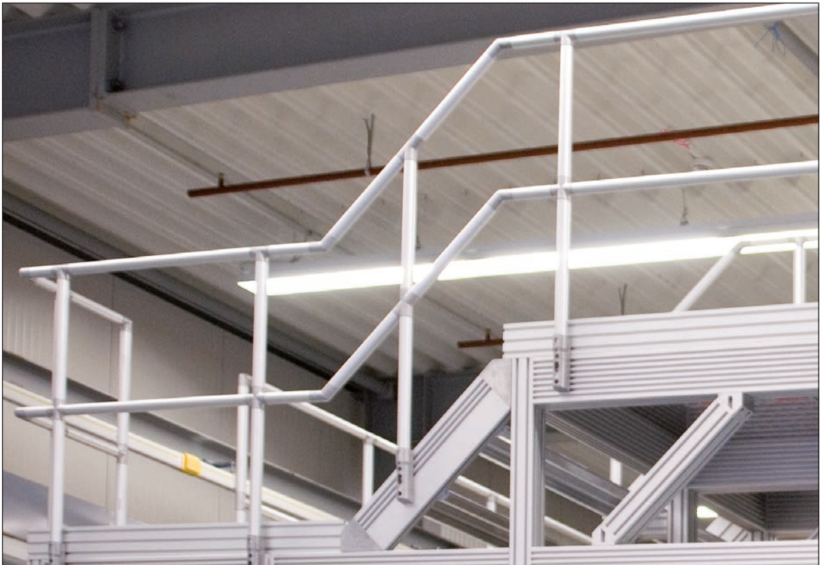
Staircase between two operating platforms.
